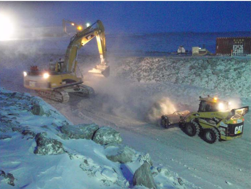
Photo 4: Bobcat with brush and excavator cleaning key trench from ~ 1+00 to 1+17, ~ E view.
