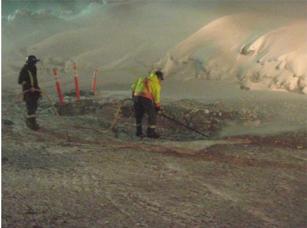
Photo 1: Compressed air blow hose being used to clean around the removed sump location (around station 0+85).
