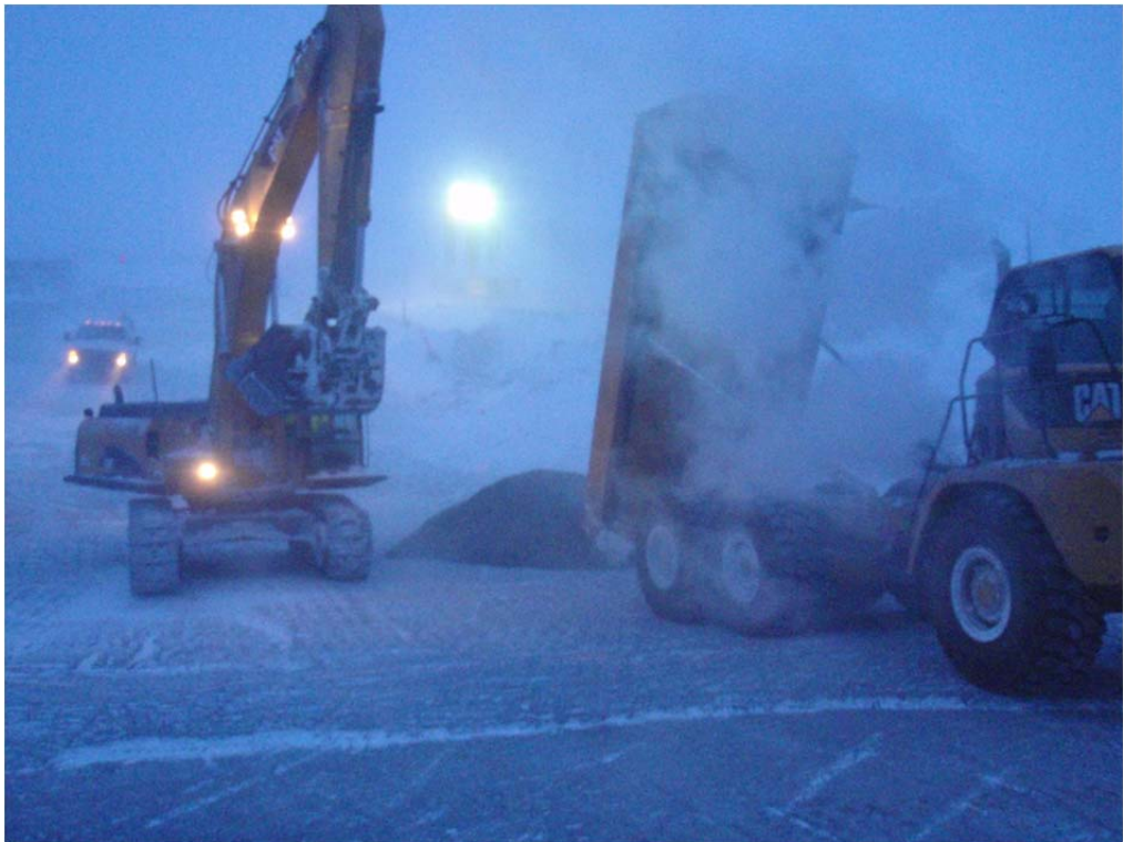
Photo 5: ~ E view of FCM starting to be placed around, 0+85 over frozen lift placed on 2012/01/15.
