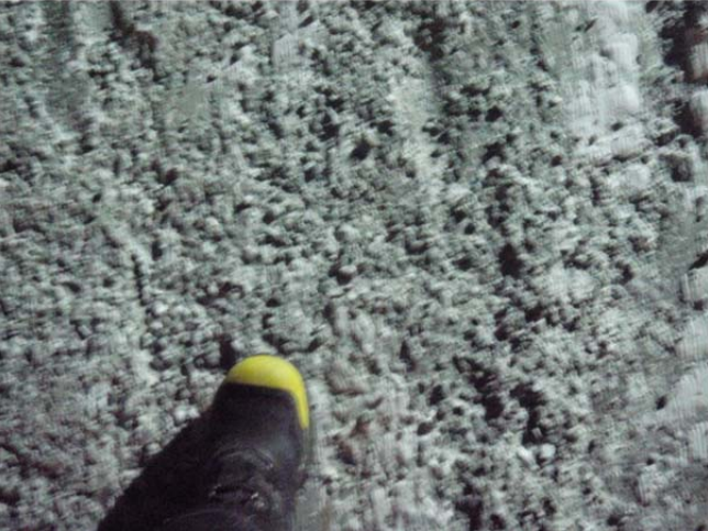
Photo 3: Close up view of surface cleaning around station 0+50. Note that frozen and loose 5/8" material is observed at this surface. This area required further scraping (likely with an excavator with a finishing bucket) before approval for placement. Note that the 5/8" material higher on the slope is less saturated and not incorporated into the FCM like it was observed to be in the central area.
