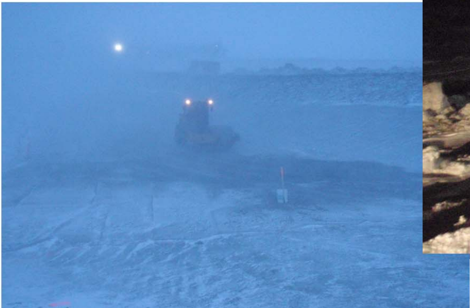
Photo 10: View of FCM placed today around the central portion of the key trench ~ 0+80 to 1+00. Note that conditions are progressing towards 'white out'.
