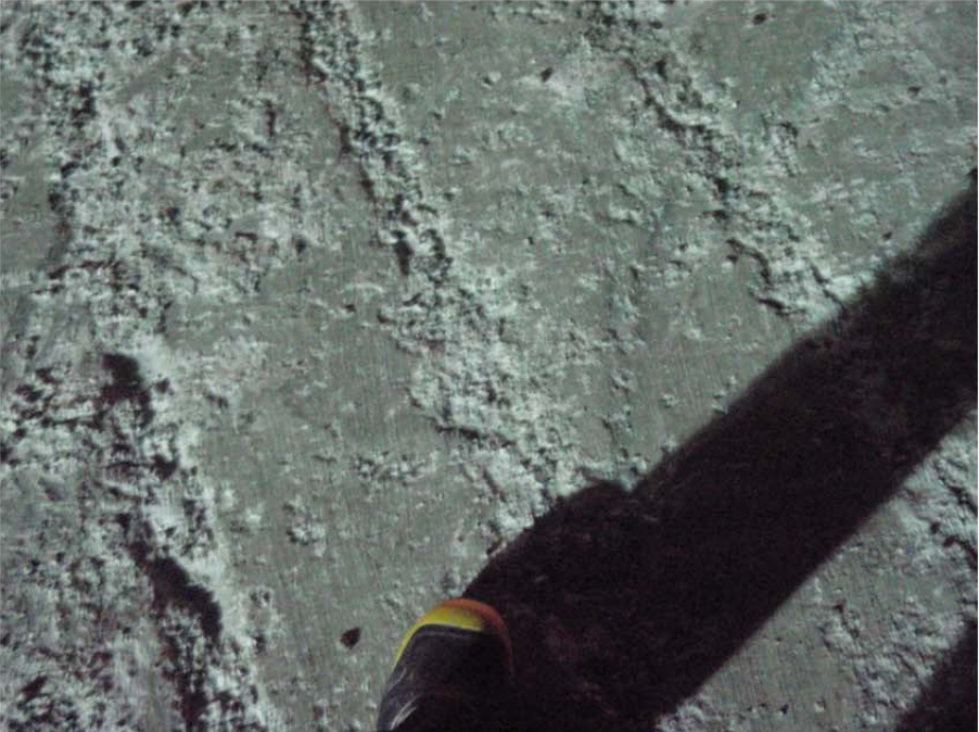
Photo 2: Close up view of surface cleaning around station 0+60. Note that this 2011 frozen core can be observed at this surface. This area is near a grade acceptable for placement.
