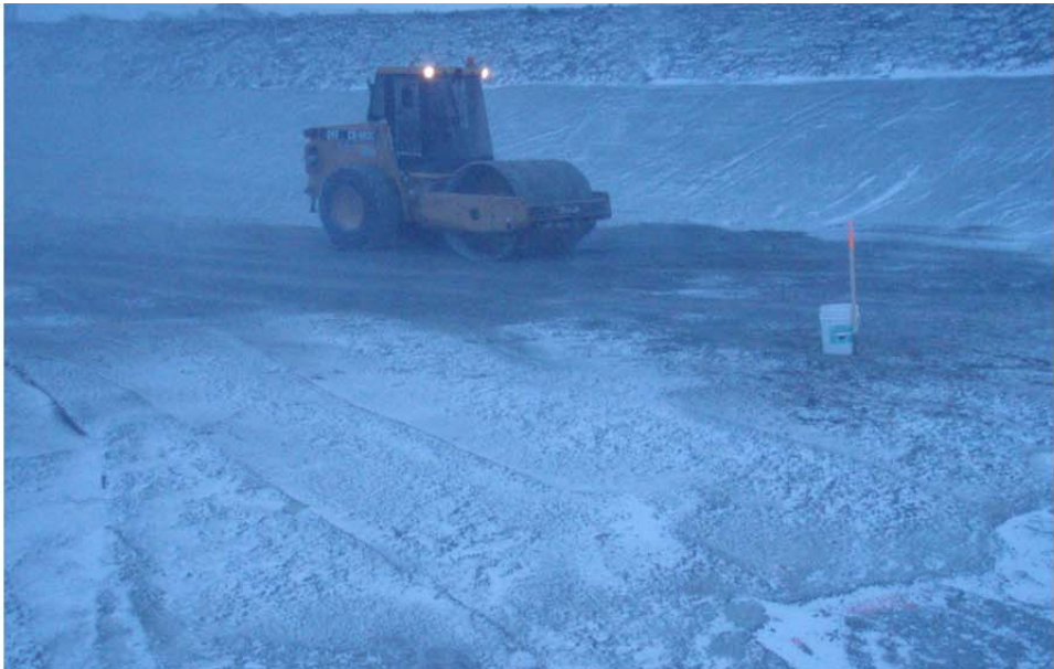
Photo 9: Smooth drum vibratory compactor packing FCM around the inflection point of the key trench. Note the installed single bead thermistor in the white bucket.
