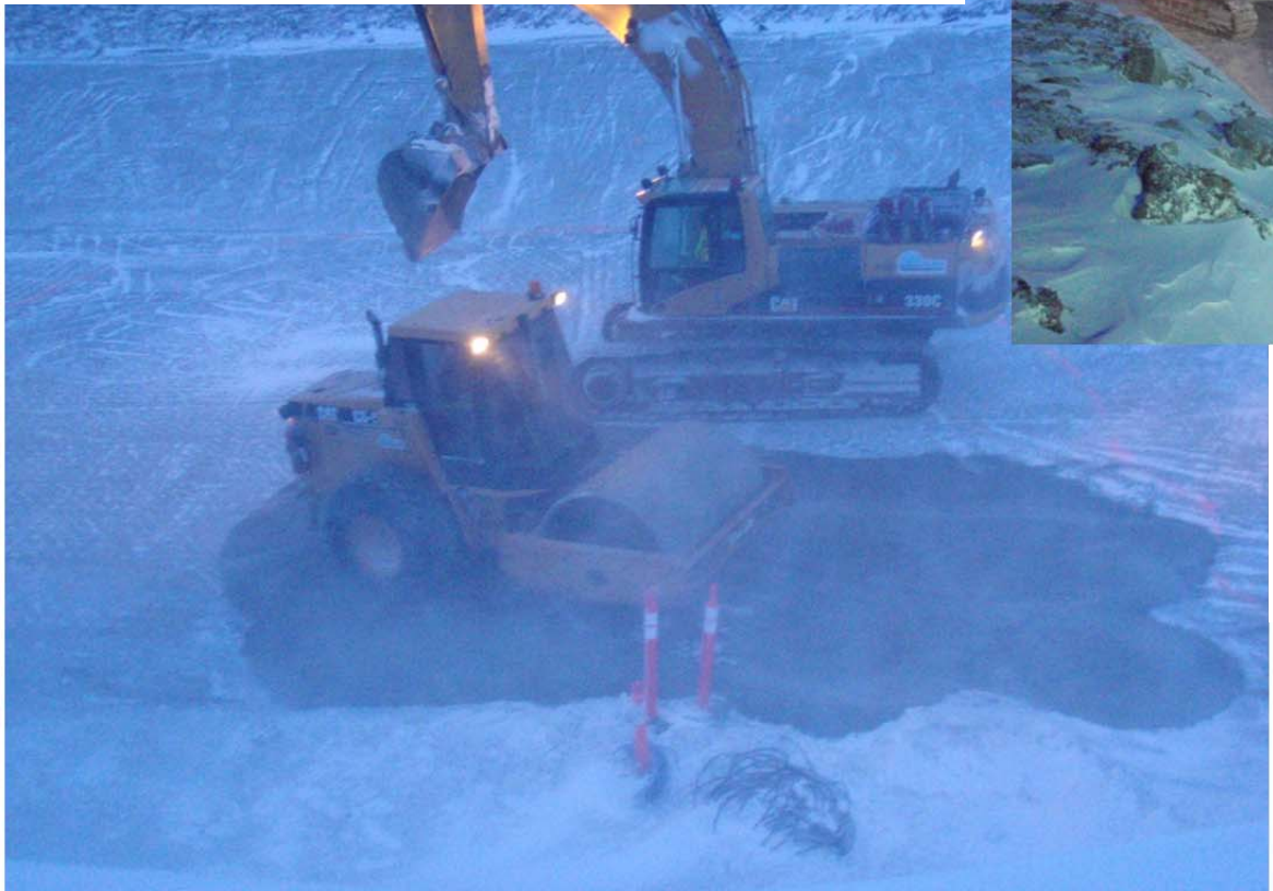
Photo 6: Smooth drum compacting FCM, placed by the 330C excavator around station 0+80 to 0+90, ~ ESE view.
